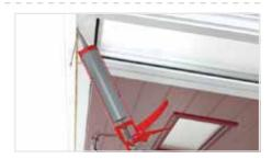
Apply the selected capping intumescent mastic in the (minimum) 10mm deep void on both sides of the doorset. Cap over the face of the any exposed packers.
